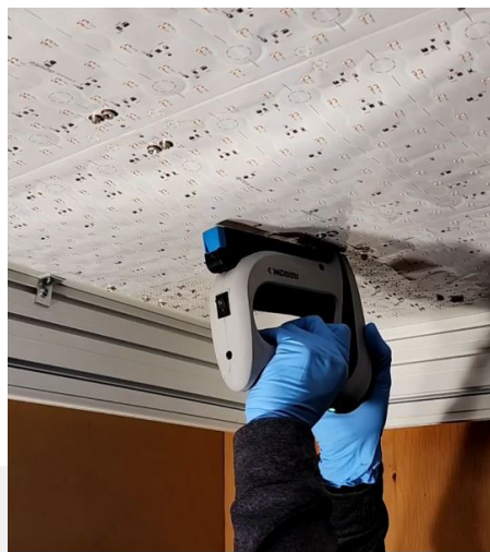
TILE INSTALLATION (EC or COOLEDGE)
