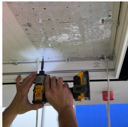
TILE INSTALLATION (EC or COOLEDGE)
