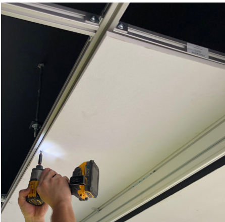
BACK PANEL INSTALLATION (COOLEDGE)
